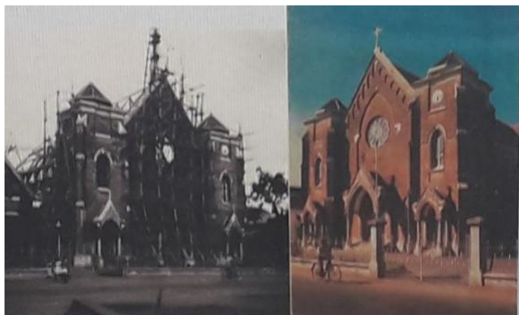
Picture 3, The church's condition during and after renovation
